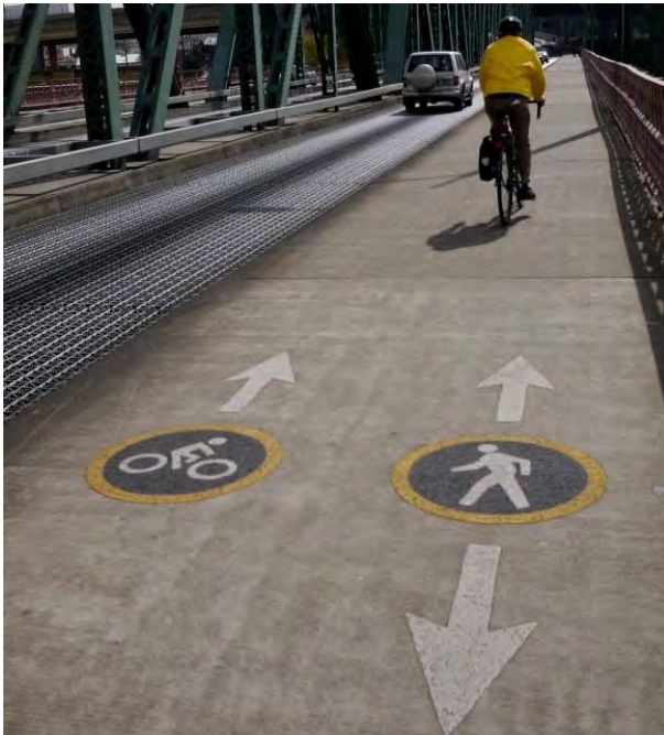
Figure 2. Example showing colored/textured pavement used to demarcate bike and pedestrian travel ways (Brazil)
